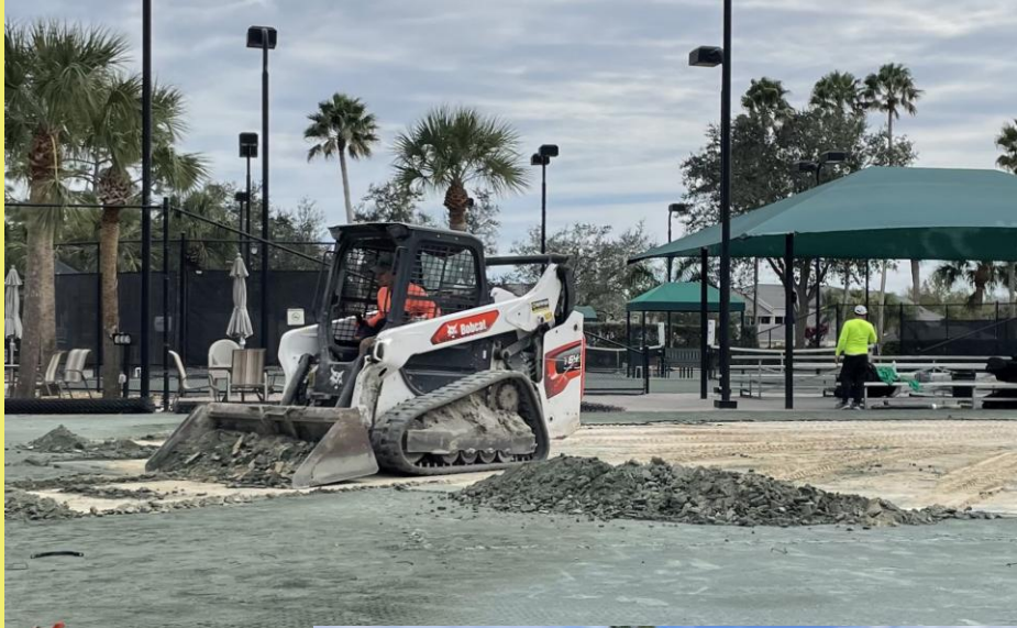
Scraping the clay off of the existing tennis court.
