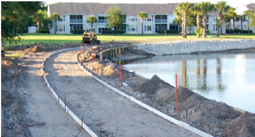
#16 - Cart path formed & bulkhead built
