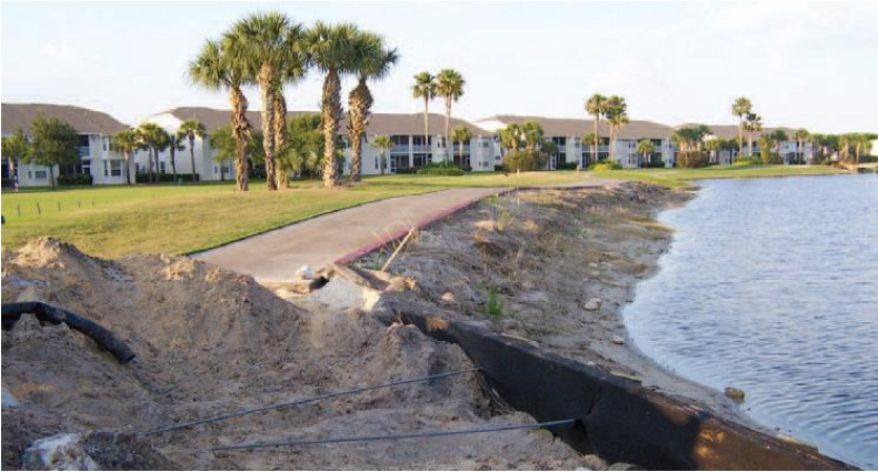
Royal 16 - Removing cart path & building bulkhead
