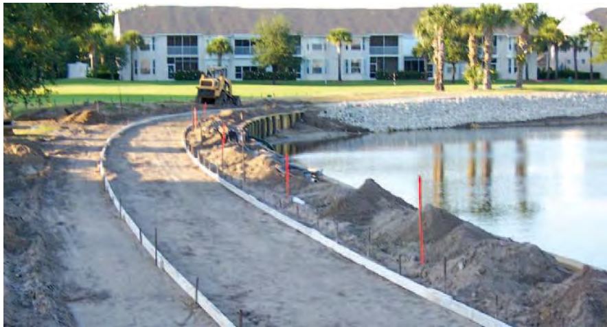
#16 - Cart path formed & bulkhead built
