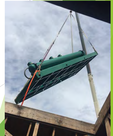
Crane install of skid.
