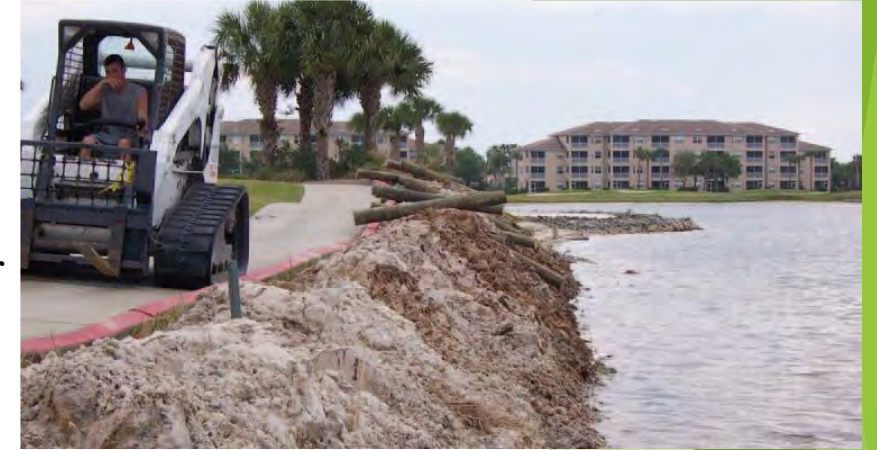
#17 - Preparing shoreline for bulkhead installation
