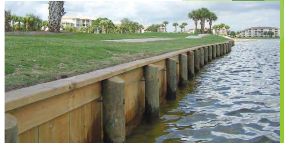
#17 - 370 feet of bulkhead with additional fairway extension
