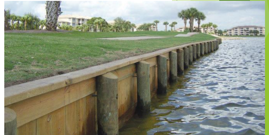
Royal 17 - 370 feet of bulkhead with additional fairway extension
