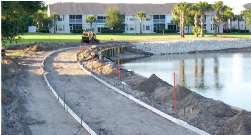
Royal 16 - Cart path formed & bulkhead built
