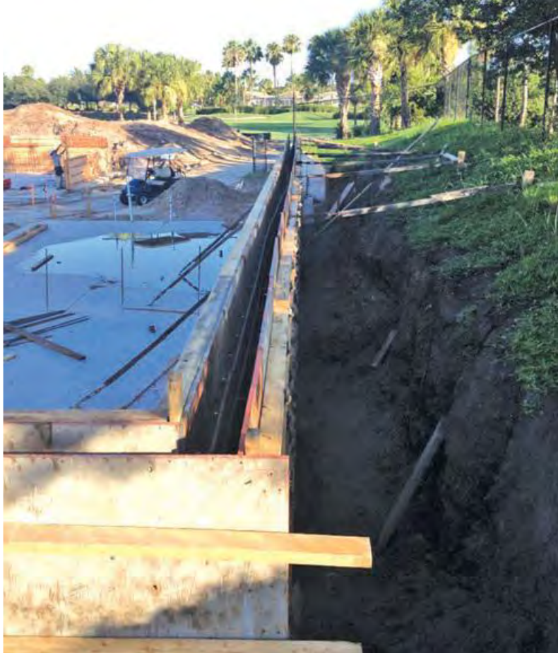
Forms for the new chemical and fertilizer storage room.
