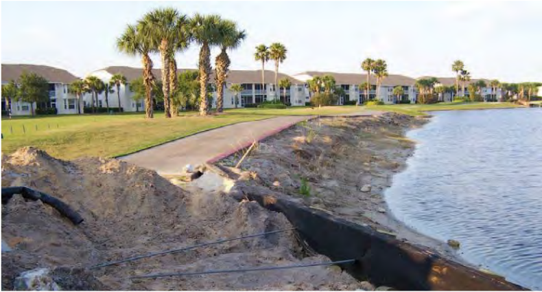
#16 - Removing cart path & building bulkhead
