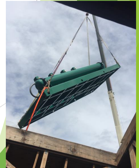
Crane install of skid.
