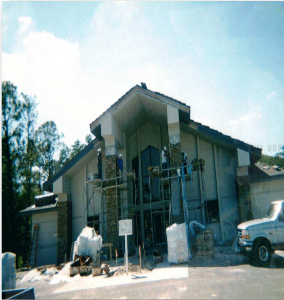
Lodge and Tiki Bar under construction 2001
