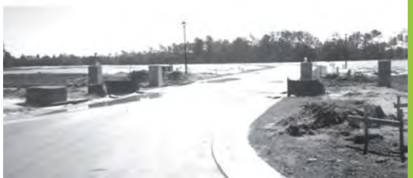
Initial construction of the Enclave entrance.
