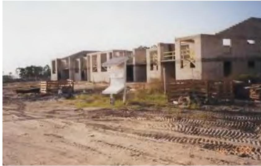
Construction of Verandas on Queen Palm Lane in October, 1998
