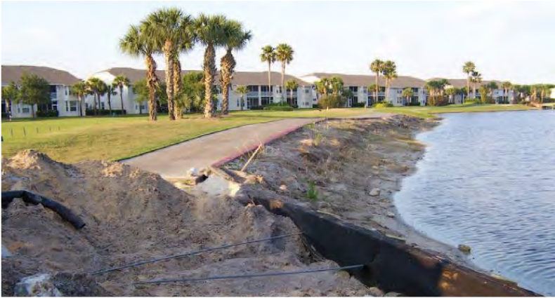
#16 - Removing cart path & building bulkhead
